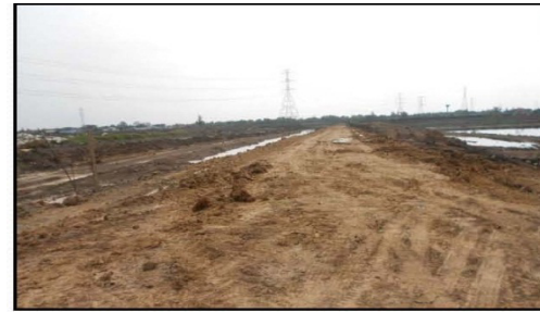
Fill Embankment & compact El.+2.90m.
