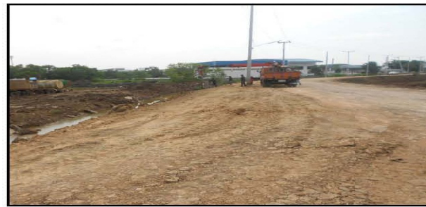
Fill Embankment & compact El.+3.70 m.
