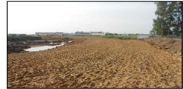
Fill Embankment & compact El.+2+60m.
