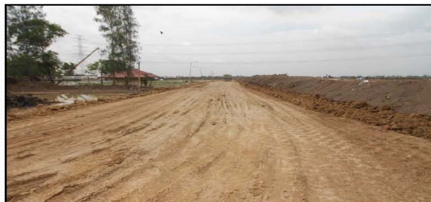
Fill Embankment & compact El.+2+50m.
