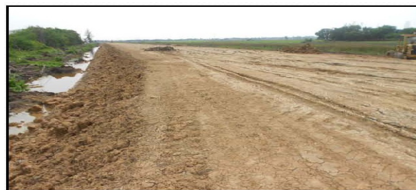
Fill Embankment & compact El.+3.90m.
