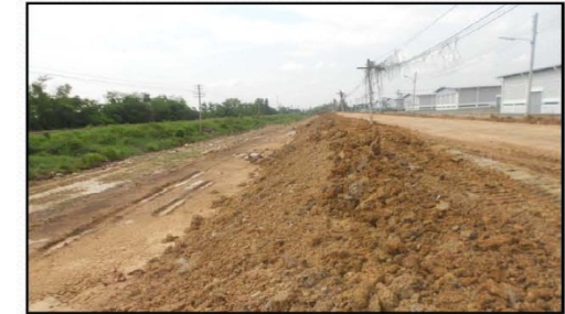
Fill Embankment and compaction El.+4.30 m.
