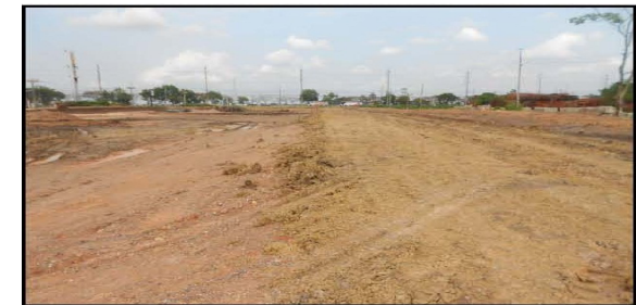
Fill Embankment & compact El.+3.70 m.
